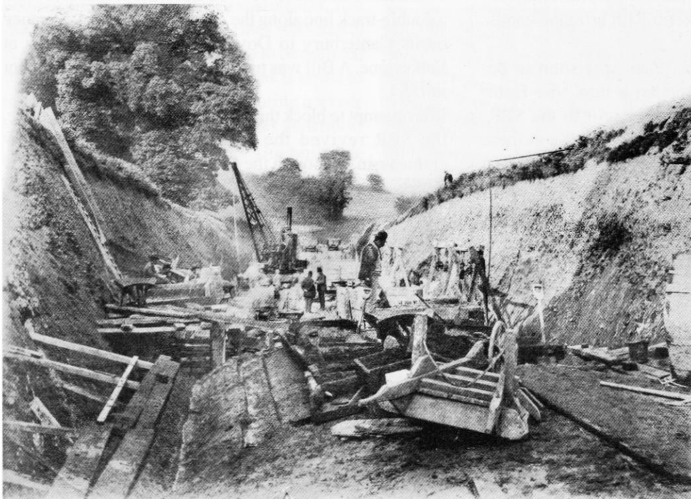
Looking north from the roof of the cut-and-cover tunnel at Bourne Park during construction in 1888. Photo from Brian Hart collection
